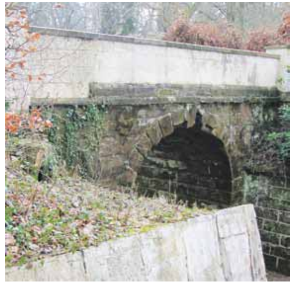
Sandstone bridge, Hewell Park
